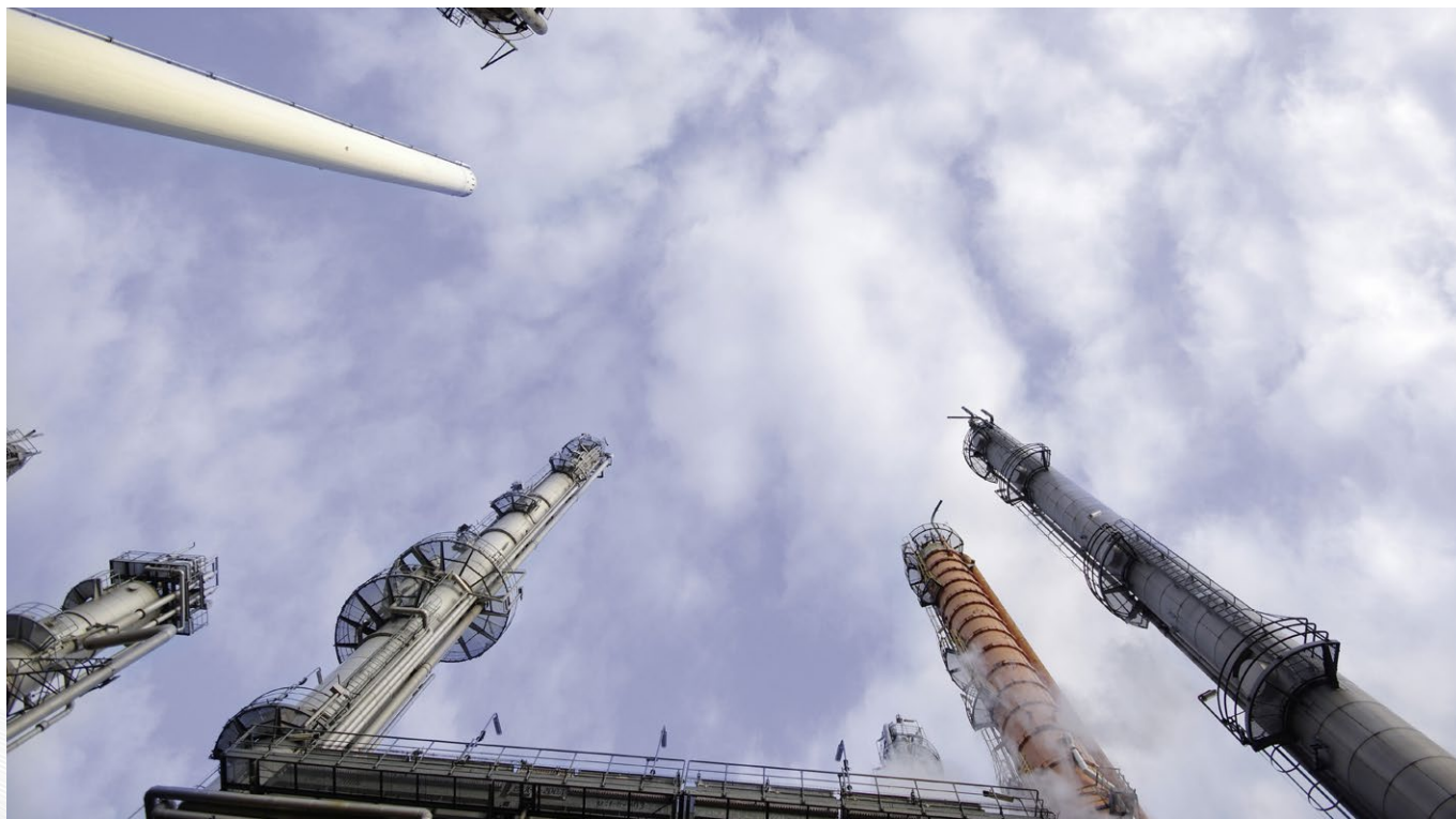
Chimneys of the Holborn refinery in Hamburg-Harburg.
