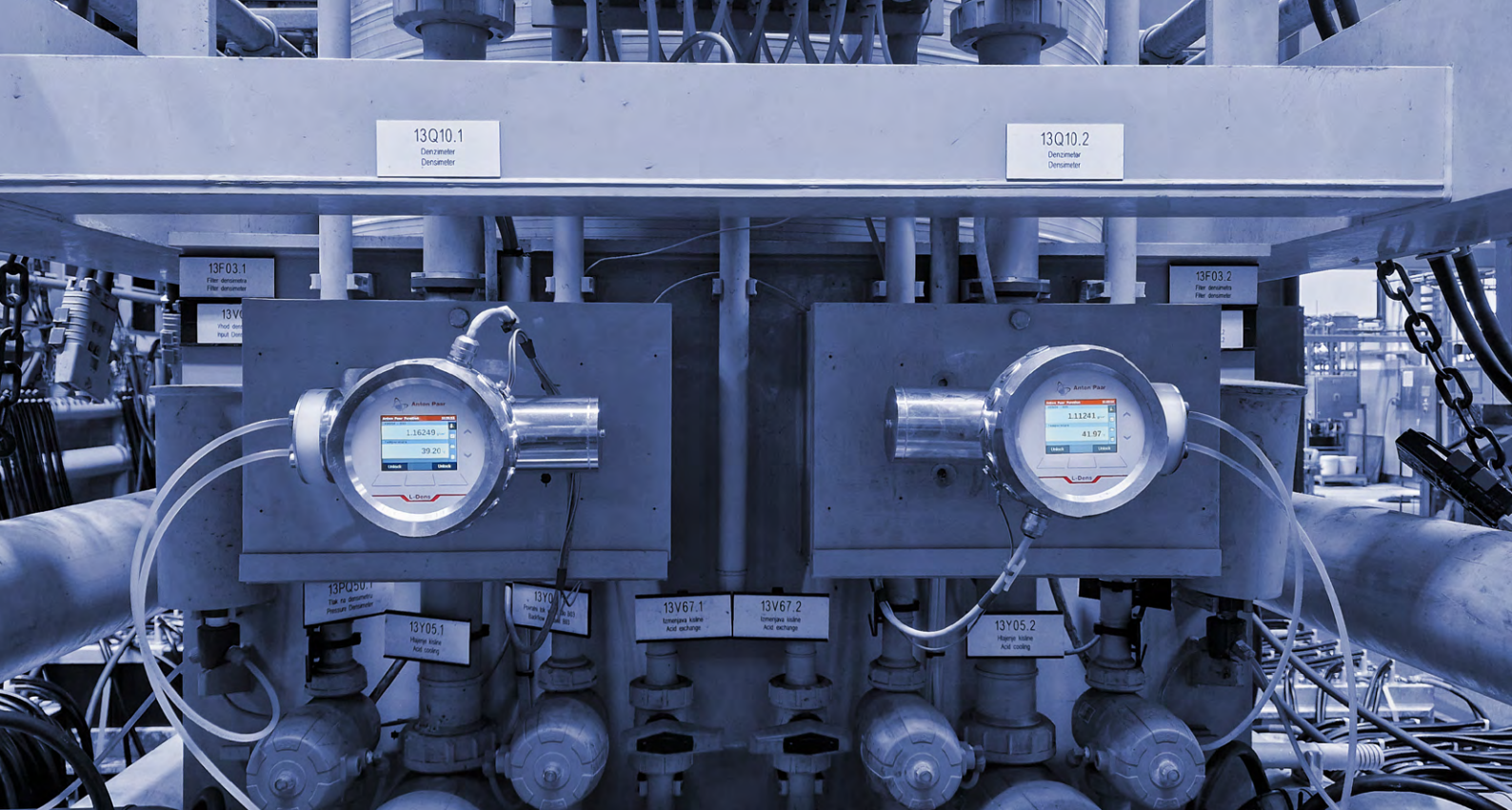
→ Anton Paar L-Dens 7400 sensors installed at TAB in Slovenia.
